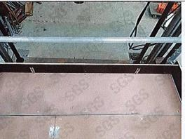
Installation details for toe-board
